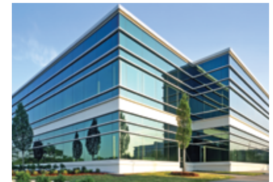
Alpharetta Center Curtain Walls
