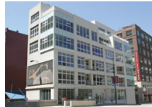
400 Orleans Chicago Window Walls
