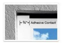
2. Ensure the trim has not been compromised by being coiled for extended periods of time and that the adhesive hasn't been exposed to direct sunlight. These types of circumstances can cause the trim to fail. If the trim has been coiled, lay it in the sun, adhesive-side down, allowing the trim to become pliable and retake its' original form.
