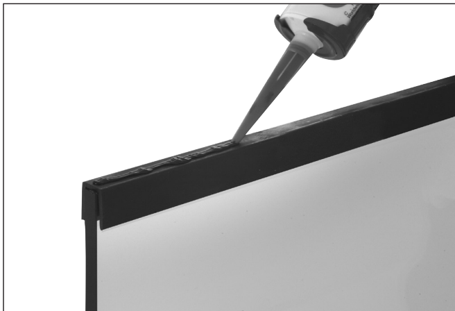
Apply Silicone to the top edge of the Protective Vinyl Insert.
