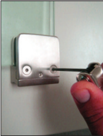
First, loosen the Flat Head Screws
