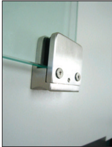
Loosen enough so the Screw Heads project above the Clamp
