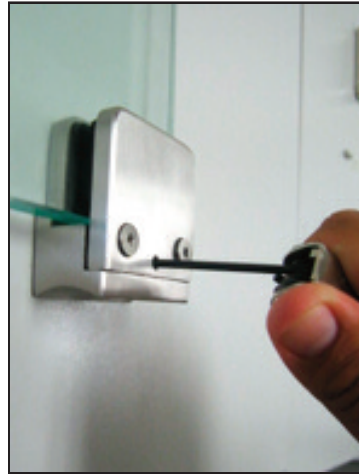
Then slightly tighten the Allen Screw so the Plate tilts at a slant.
