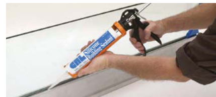
Gun Cap Bead of Silicone
