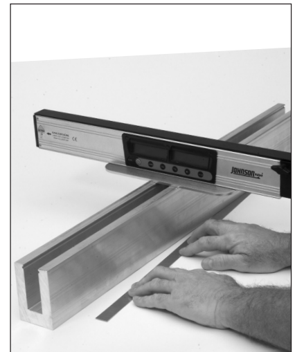
Use the "PAL" Tool to assure the Base Shoe is level at all points. When leveling the Base Shoe make sure you level the shoe within 0.4 degrees of the floor. Angular variation up to 0.4 degrees is acceptable during this process.
