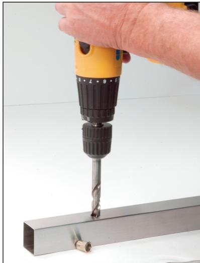
First, drill the appropriate size hole for the Rivet-Nut into your round post or square tube
