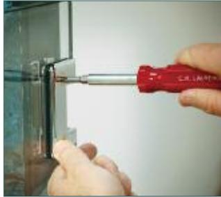
After alignment, tighten the cover plate screws by hand. Do not use a power tool, or you risk damaging the screw heads.
