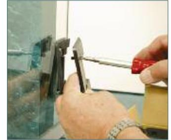
Install a new gasket and interior cover plate, replace screws, then secure in place.
