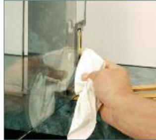
Block the door to maintain alignment and remove the cover plate. Clean glass in gasket area.
