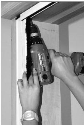
Diagram 10 - Attaching Top into Header
