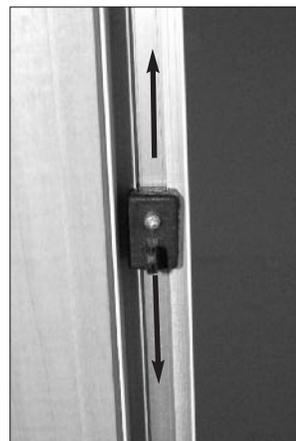
Diagram 12 - Adjusting Plastic Hook Latch
