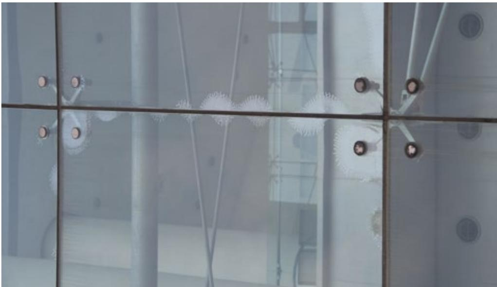
Typical defects caused by delamination.
