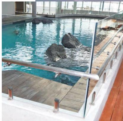
CRL One-Piece Clamps, (AFWC1) are designed for insertion in core-drilled holes in a deck or on top of a wall. Glass fabrication requires two 3/4" (19 mm) holes per Clamp. Height: 9-13/16" (250 mm).
