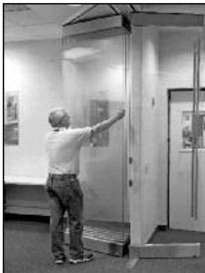
Fig. 1 Beginning to extend the panels by pulling the leading edge
