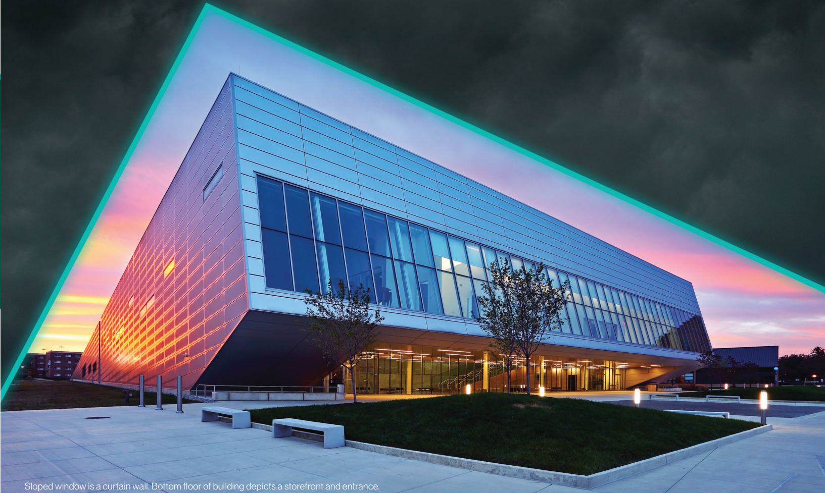
Sloped window is a curtain wall. Bottom floor of building depicts a storefront and entrance.
