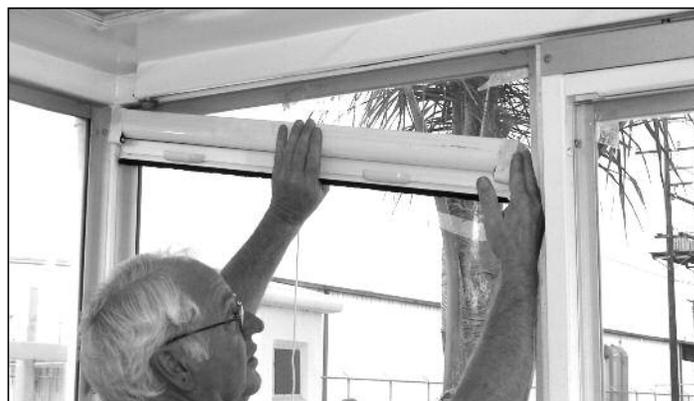
**STEP 8** - Slip side channel end caps onto side channel. Position pull bar locking cap as shown.
