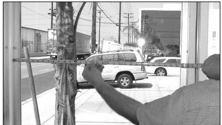
**STEP 3** - Measure the cassette including the existing end cap, and mark the cassette for cutting at 1/4" (6.4 mm) shorter than the measured inside jamb width opening. Holding the pull bar (B) tight against the cassette (A), cut the cassette, pull bar and screen cloth evenly all at the same time. Note: Due to the length of the torsion spring inside of the cassette, the minimum window opening width is 24" (635 mm).
