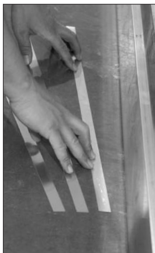
Slide Shim Strips under Base Shoe to fill gaps
