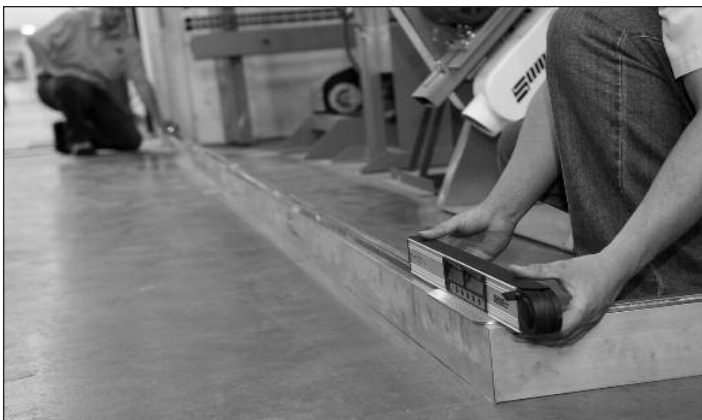
Align the "PAL" Tool with base shoe and point toward the Laser Target set at other end of base shoe
