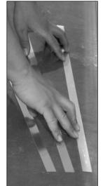
Slide Shim Strips under Base Shoe to fill gaps.
