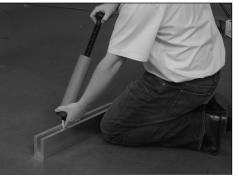
Step 3 Install CRL's Expansion Bolt Concrete Anchors.
