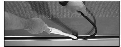
**For Exterior Applications:** Use CRL's BSG250 Fast Seal Glazing Vinyl for glass railing applications where there is no access to the outside shoe edge. It's designed to be installed to the outside cladding edge before the glass is set in place, eliminating the difficulty and risk of reaching over the guard rail for seal installation. Use CRL's BSG100 or BSG500 Roll-In Glazing Gasket to finish off top inside edge of the base shoe pocket.
