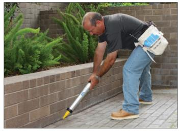
Construction Polyurethanes for concrete-to-concrete expansion joints in tilt-ups, and other masonry joints.
