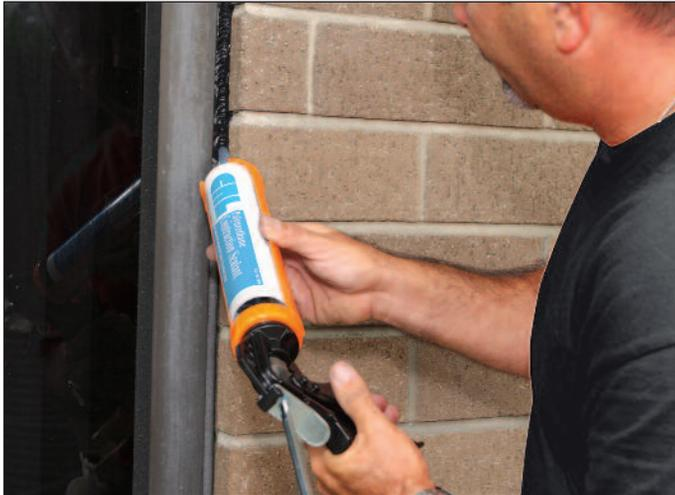
Construction Polyurethanes for metal-to-concrete/brick storefronts, and residential vinyl window perimeter sealing.
